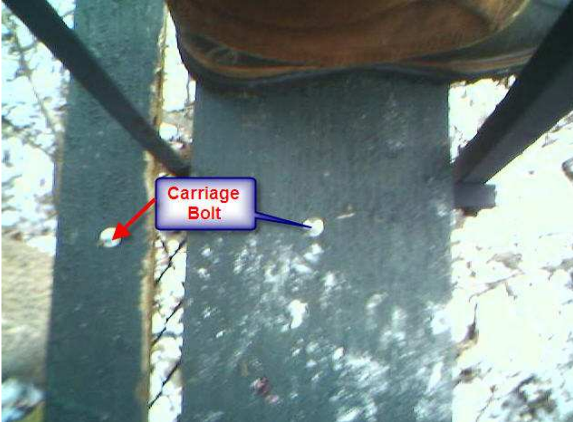
Figure 3. Left foot on a Wing, carriage bolts
