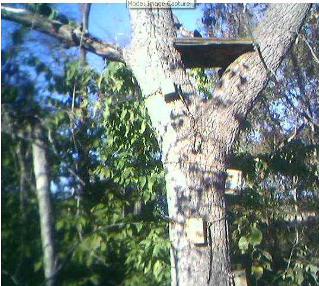
Figure 7. Y-board Tree Stand with 4x4 steps.
